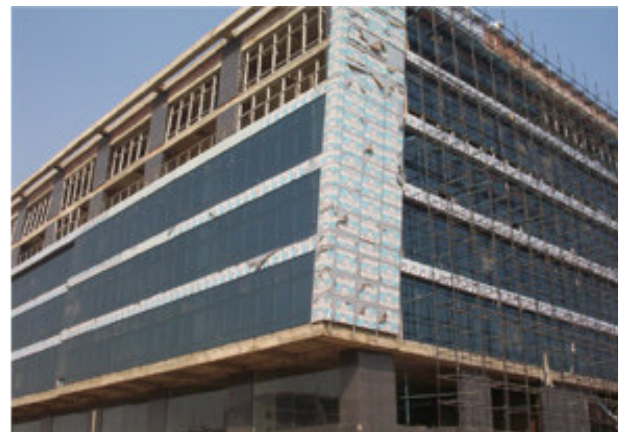
Aditya Building, Jasola District Center, South Delhi.
